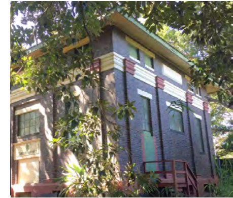
The pleasing proportions of Substation No 5, designed by R.R. Ogg, located near Newstead House.
