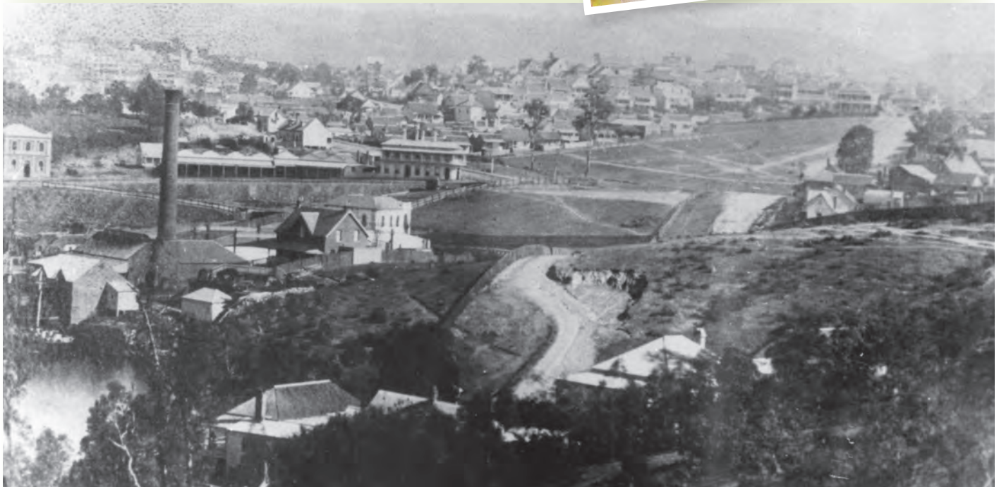
On the Boundary: A view ca 1880, probably from Bowen Tce, of Petrie Bight in the left foreground, with Boundary St heading up towards St Paul's Tce. Near the centre of the image is the Hotel Orient dating from 1875. (QUT Digital Collections)
