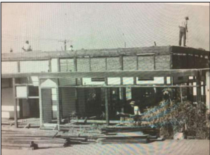
Deconstruction of Japanese House for transportation to Ingham
