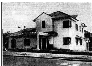
1 Oxlade Drive, photo from BCC Brisbane Heritage Register
