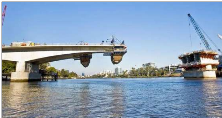
The Go Between Bridge under construction
