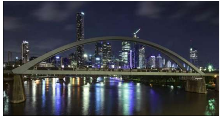
The double arches of the Merivale Rail Bridge
